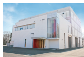
Photo 1 Fire Research and Test Laboratory
