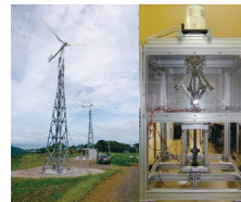
Monitoring of output power from multiple small wind turbines, and a prototype of a flywheel energy storage system
