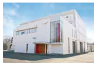
Photo 1 Fire Research and Test Laboratory
